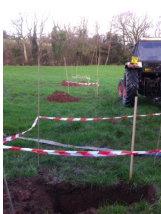
All 3 pits on Feb 10, 2016
