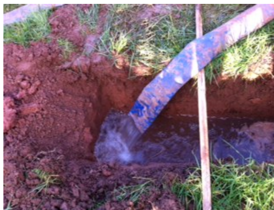
Filling pit 1 on Feb 10, 2016
